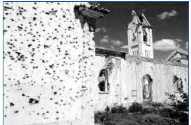
A bullet-scarred church in Kuito, Angola. The country's decades-long war was fuelled in part by oil and diamond revenues. Foreign oil companies, mostly offshore, continued to operate profitably. (Photo: Africaphotos.com)
